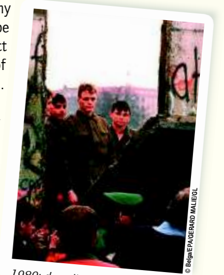
1989: demolishing the Berlin Wall.
